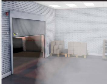
Often in conjunction with an integrated ventilation system, smoke compartments are formed to prevent smoke spreading throughout a building. They must be impermeable to smoke leakage, within set criteria, but also offer a level of resistance to heat.
