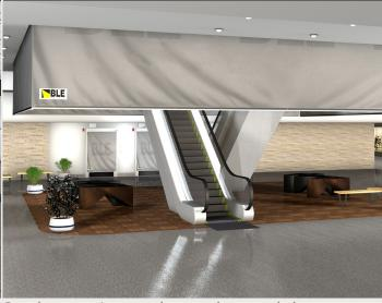
lower level to create a deep reservoir to prevent smoke moving to upper levels. Fire curtains can be used to seal off the stairwell completely if required. Intelligent control systems linked to the escalator operation can be provided to ensure effective means of escape are maintained.
