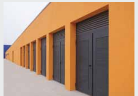
⑨ Multipurpose Doors
